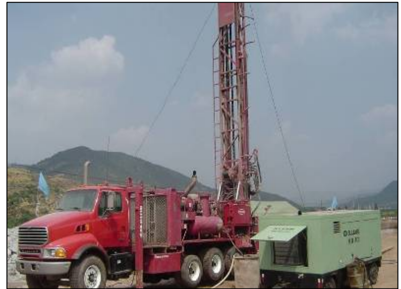
Mobile drilling rig
